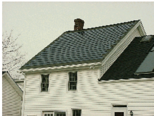
SolarOptions first net-metered customer with a 2.7 kW Sunslate™ system received an $8,256 rebate check.
